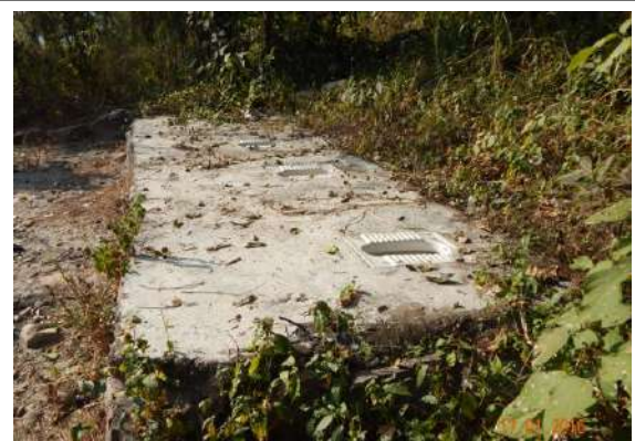
Permanent toilet structure
