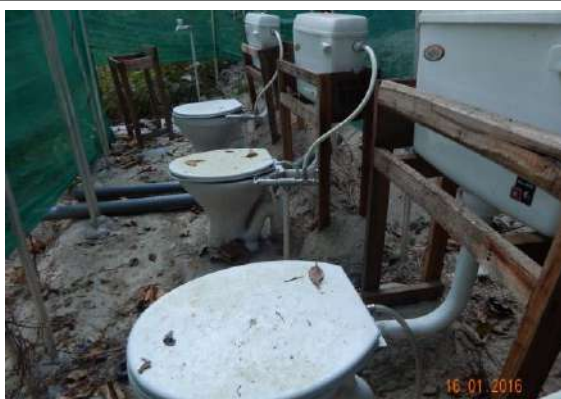
Permanent toilet structure
