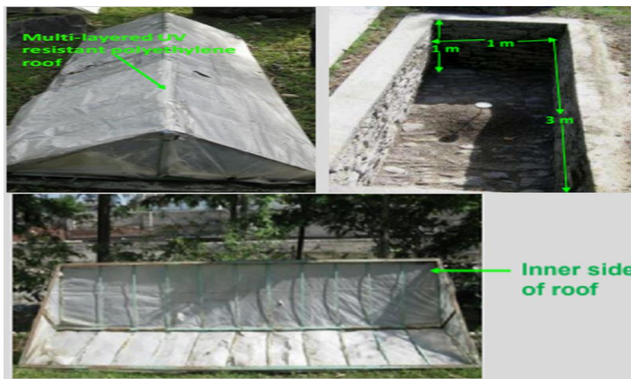
Fig. 7. Structure and design of microbial composting pit
