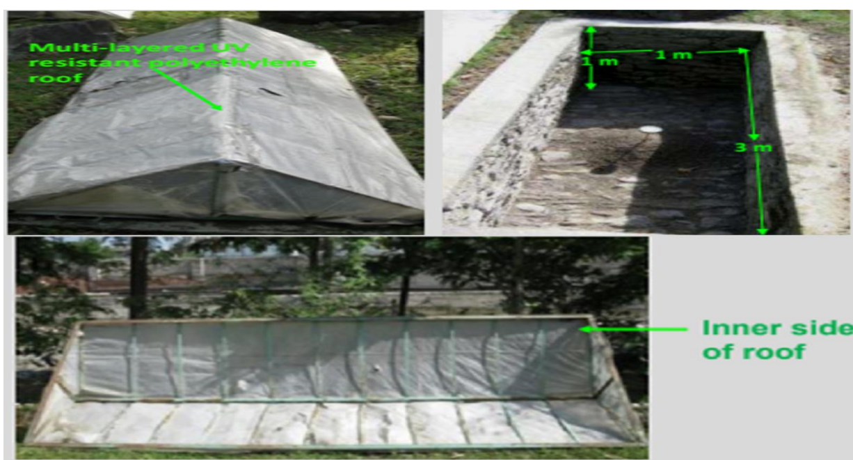
Fig. 4. Structure and design of microbial composting pit
