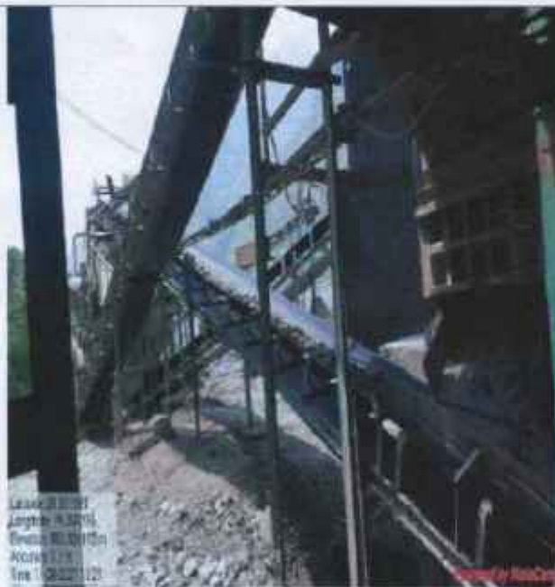
Uncover conveyor belt
